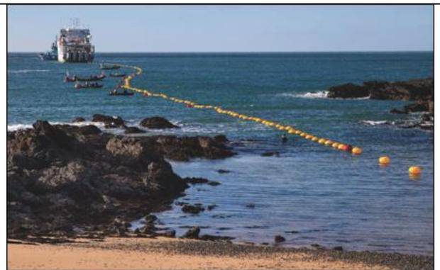
(b) Small boat fleet manoeuvring floated cable
